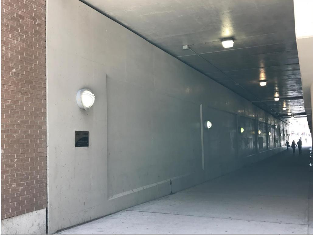
View of west side retaining wall, 73m long and 4.4m high:
