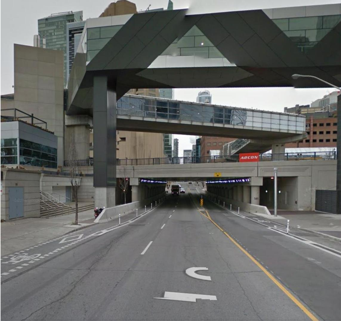
View of east side retaining wall, 80m long and 4.4m high:
