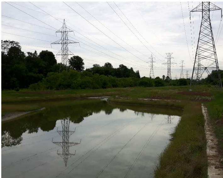
Emery Creek Pond 2 – nearing completion
